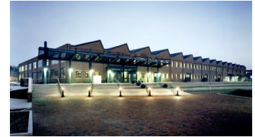
Showers Building Research And Office
