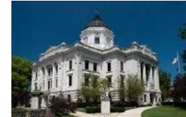
Monroe County Courthouse
