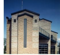
Bloomington Fire Station
