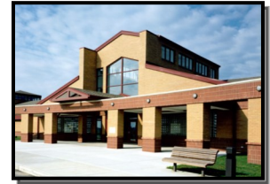
North Vermillion Elementary School
