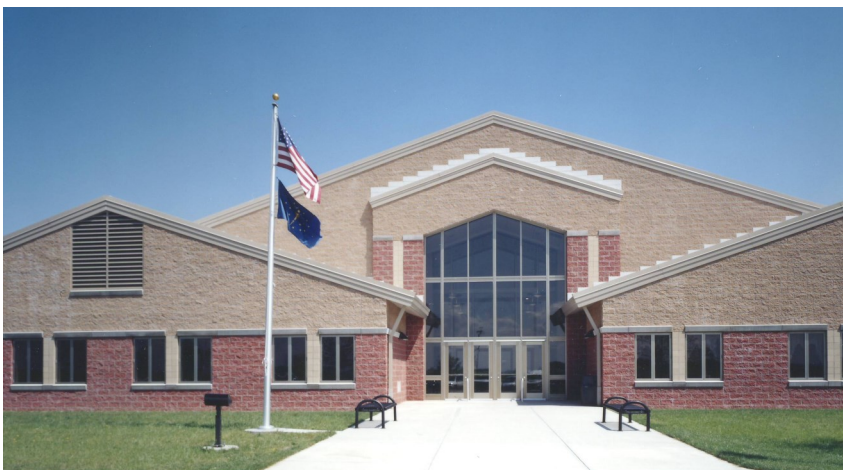
North Davies Elementary School
