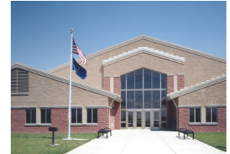
North Davies Elementary School
